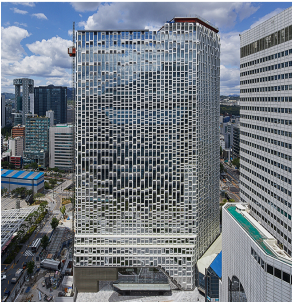
Hanwha Building's new look is an environmentally sustainable design that makes it stand out from its neighbors
