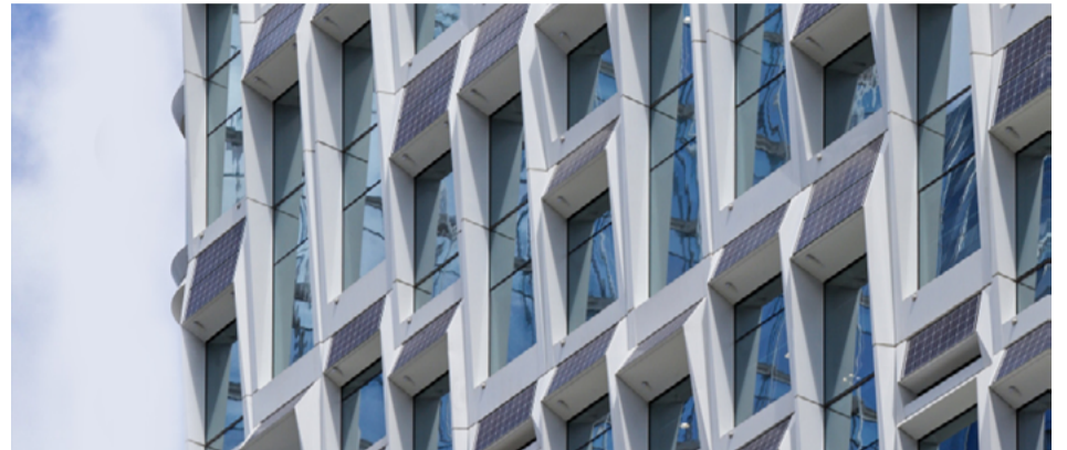
Some of Hanwha Building's window shades incorporate solar modules to produce electricity while shielding the people inside from sunlight
