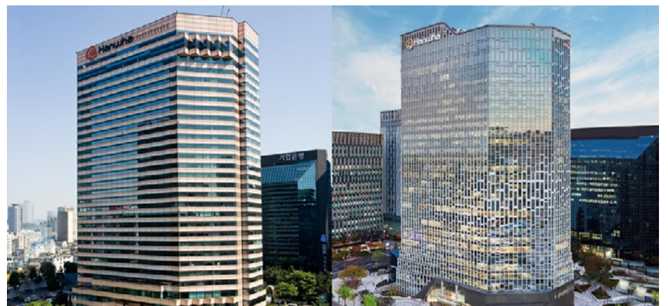
Hanwha Building was originally a standard 1980s Korean office block. Its renovation resulted in a much more distinct and dynamic look
